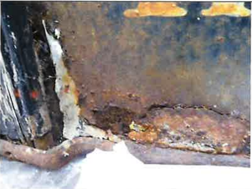
Detail of bottom left corner of side B of pub sign showing filler material between painted sign and wooden frame surround, before conservation
