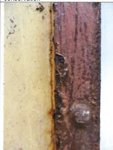
Detail of riveted steel frame at right side of side B showing disruption of painted surfaces from underlying metal corrosion, before conservation
