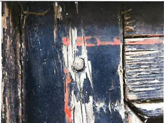
Detail of painted wooden frame surround at top left corner of side B showing wooden peg construction and red pin striping over black paint, before conservation
