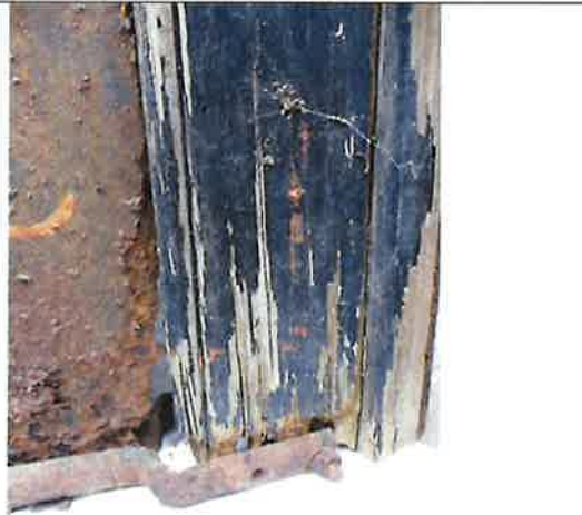
Detail of bottom edge of side B of pub sign showing corrosion through painted surfaces, before conservation
